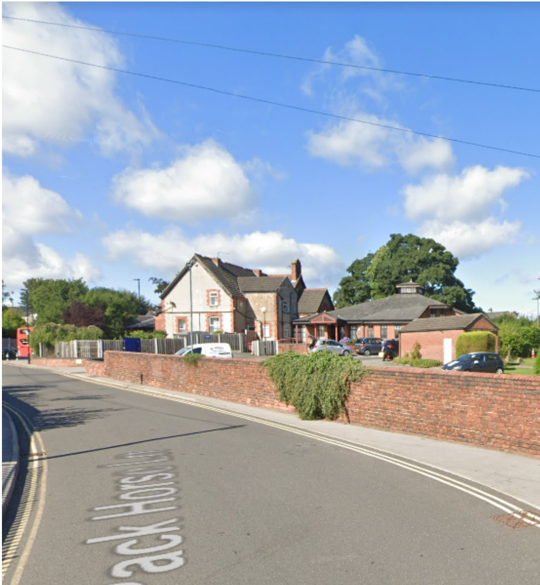
Image of T2, T3 and T4, partially visible on the right, above the roof of the church. Image taken from Google streetview from the vantage point of Pack Horse Lane.
